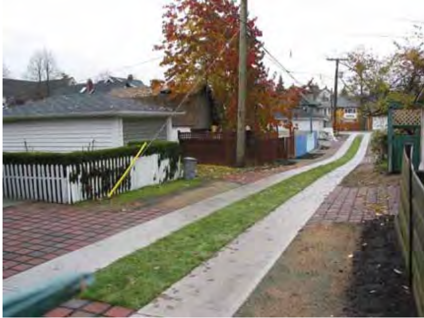
Vancouver's first Country Lane installed in 2002.
