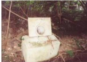
1. Dislodged/eroded drainage pipe behind Oak Summit Apartments (right bank)
