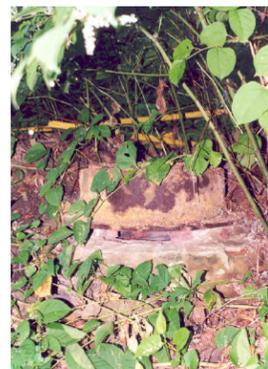
6. Broken/breached concrete collar of sanitary sewer
