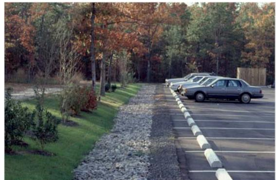
21. In areas with poorly draining soils, infiltration beds below pervious pavement may be designed to slowly discharge to adjacent wetlands or bioretention areas. Only in extreme cases (i.e. industrial sites with contaminated soils) will the aggregate bed need to be lined to prevent infiltration.
