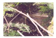
5. Broken concrete bulkhead Action/BMP: Have the township engineer assess the problem and develop solution.
